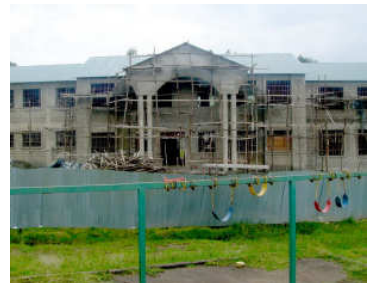
We need your help to finish the new lower school building
